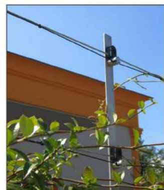
Example of L-shaped bracket with metal rope. 1 tensioning bolt every 4m.
