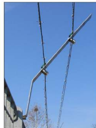
Example of overhang bracket with barbed wire. 1 tensioning bolt every 10m.
